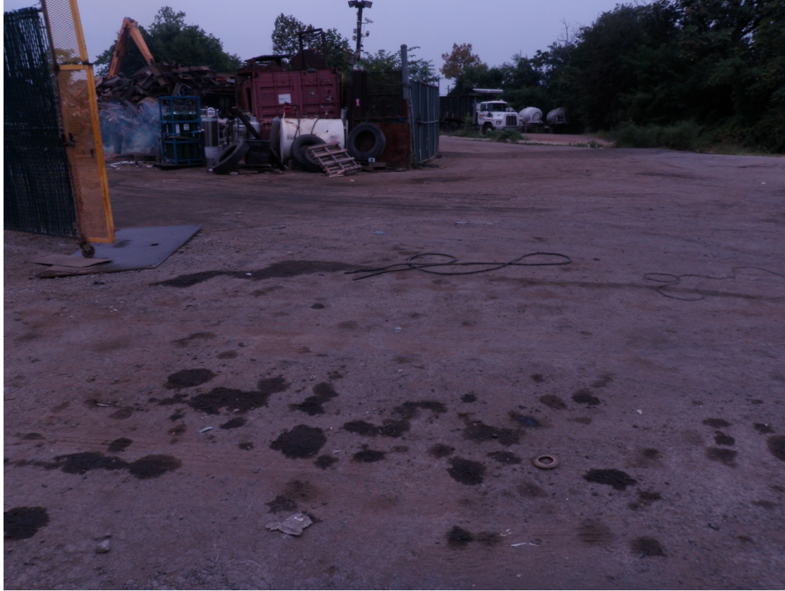
Photo #1: View of subject site from the east
