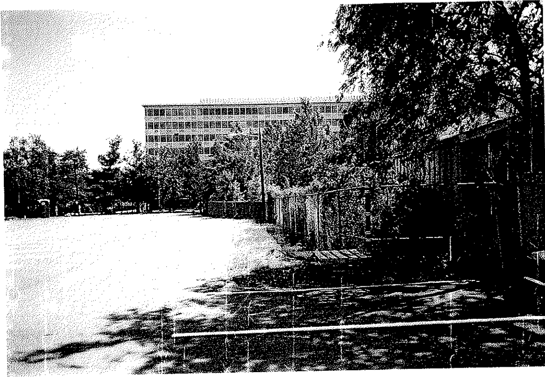
Photograph 7: View towards the southern adjacent US Coast Guard headquarters building.
