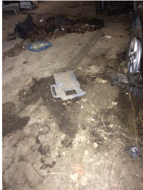
Photo #5: Staining of concrete in building
