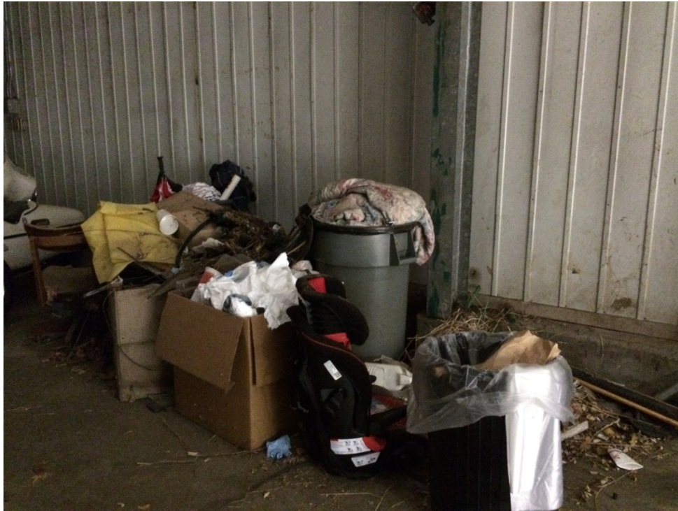
Photo #7: Storage of waste inside building
