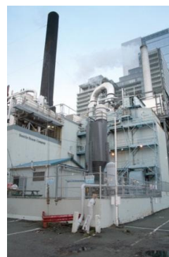
Seattle Steam Company's biomass incinerator (Photo: biomassmagazine.com)
